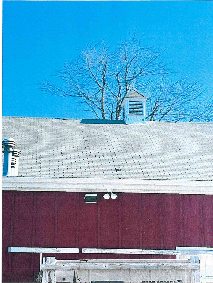
Existing Roof & Cupola
