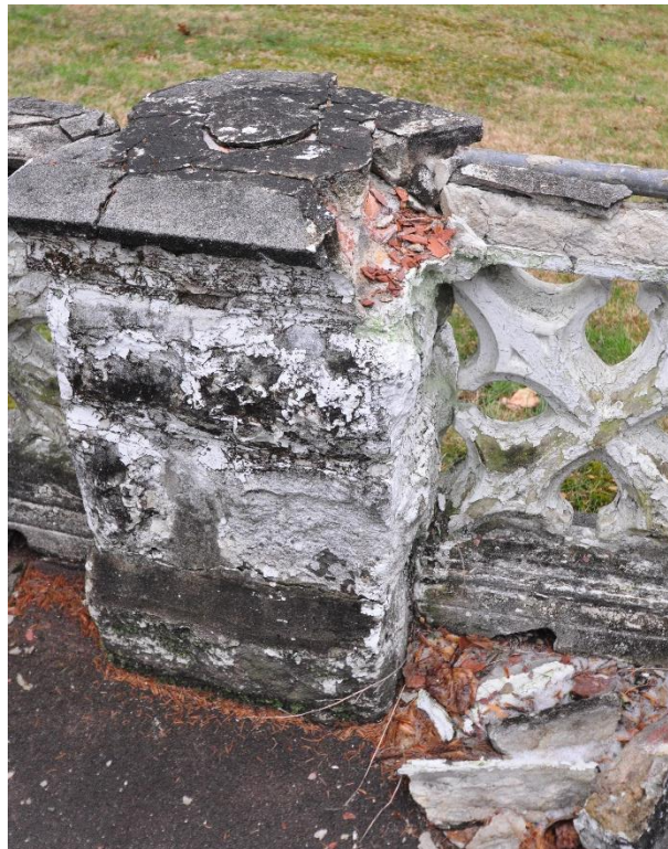
Front patio: Deteriorating masonry wall
