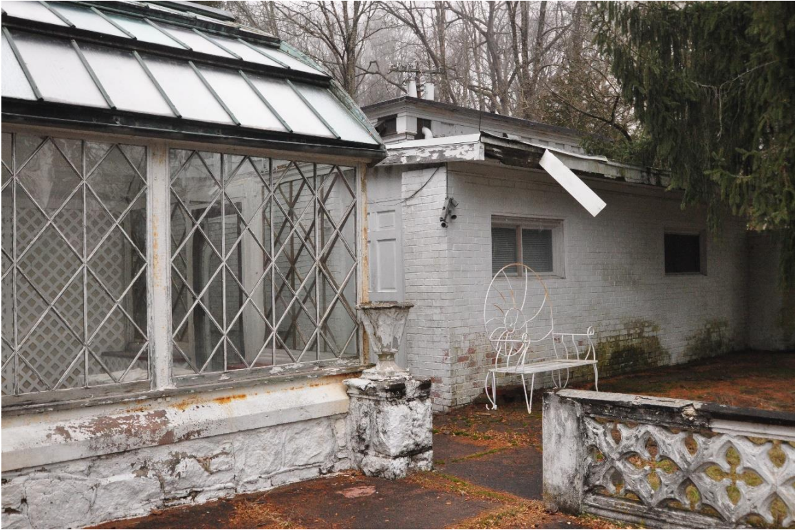
Northeastern section of building: Deteriorating conservatory, crumbling fascia, evidence of water damage, and masonry disrepair
