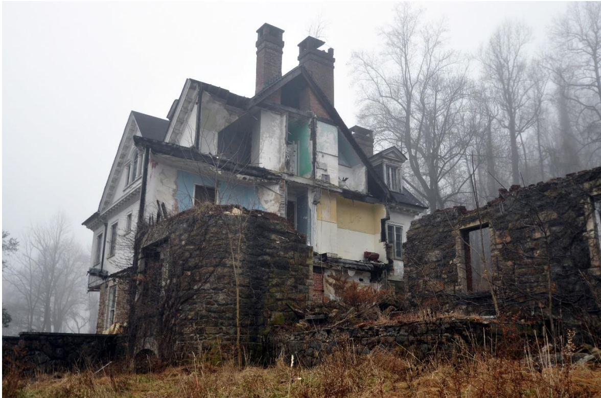
Missing eastern wing of building due to partial demolition. Also visible is the crumbling masonry/foundation wall that once supported this section of the house.
