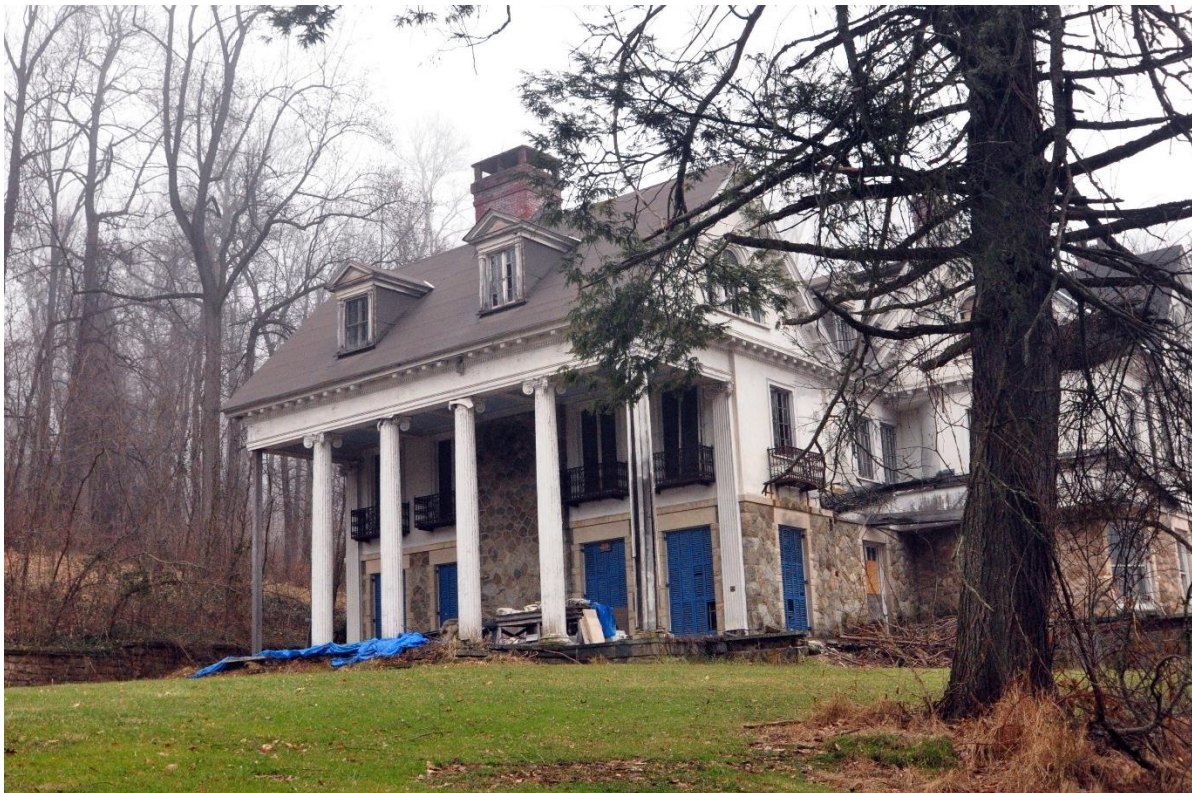
West wing of the house, showing broken windows, debris, the far left column is missing, and the far right column is in significant disrepair.
