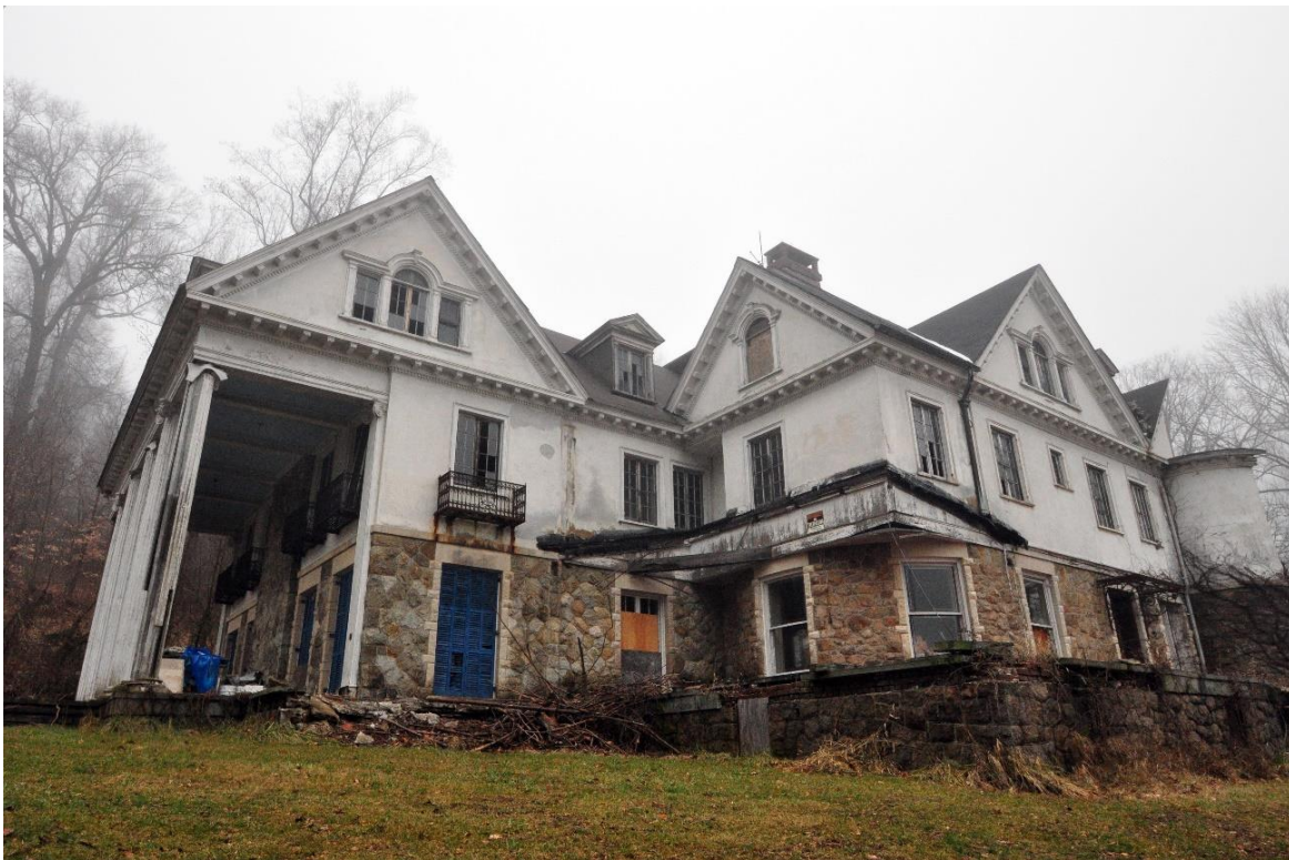
Southwest corner of structure. Visible are broken and boarded up windows, damage to the exterior wall where the roof is missing over the patio, deteriorating masonry/foundation walls, water damage.
