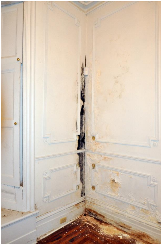
Interior: Evidence of interior water damage
